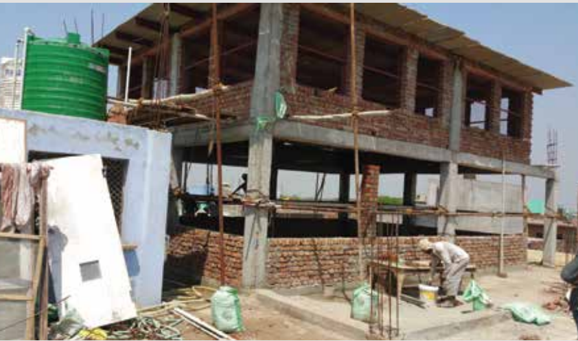
CONSTRUCTION OF MAITRI GHAR IN RADHA KUND
